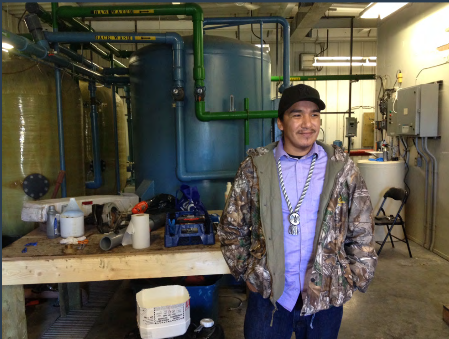
Sheldon Oskineegish in the water treatment plant in Nibinamik First Nation.
