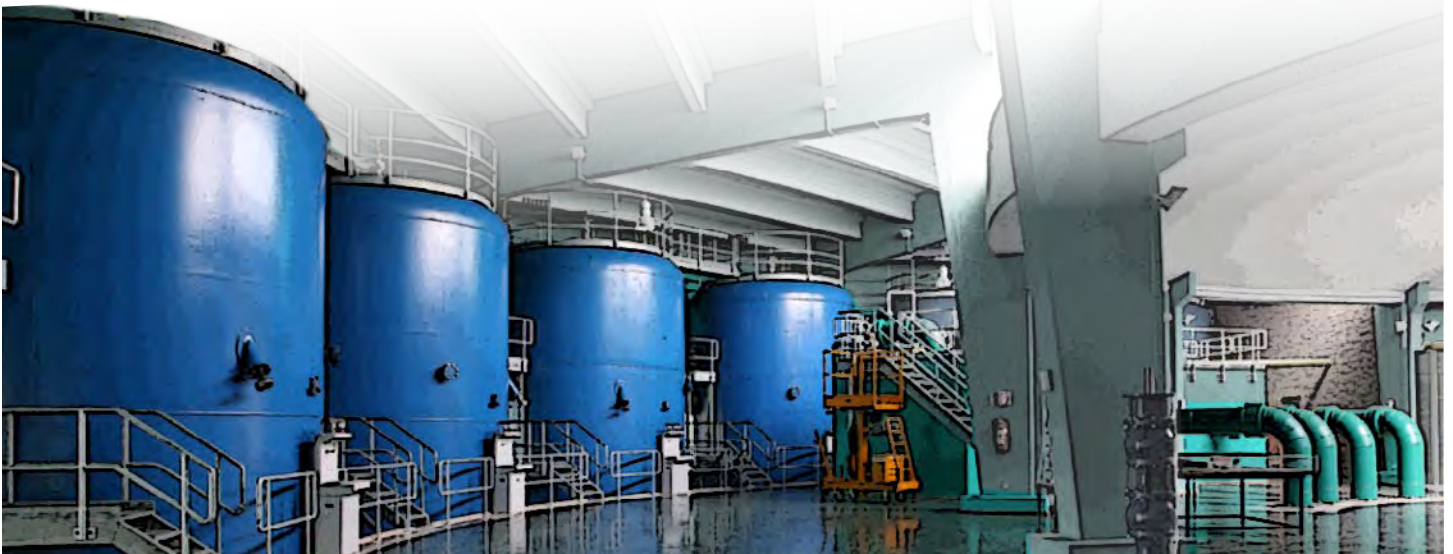
“Filterhalle Wasserwerk Am Staad” by C.Koennecke via Flickr (modified). CC by-sa 4.0
